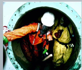
Personnel making exit from a confined space during a man-entry tank cleaning operation
