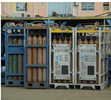
Cross-section of gaseous nitrogen & helium racks with gas cylinders
