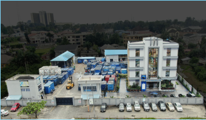
PICTORIAL VIEW OF SOME OF OUR ASSETS AT THE PORT HARCOURT BASE
