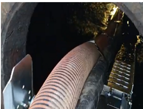
Robotic oil storage tank cleaning in action (containerized accessory unit package)
