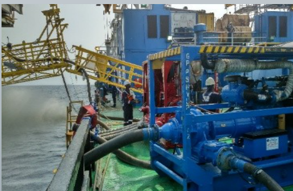
An onsite high-velocity high-volume pipeline flushing operation in progress
