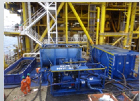
Cross-section of a velocity high-volume pipeline flushing operation in progress onsite
