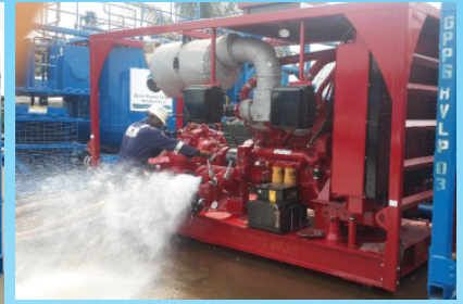
Cross-section of typical operational setup of pipeline flushing project to free the line of hydrocarbons
