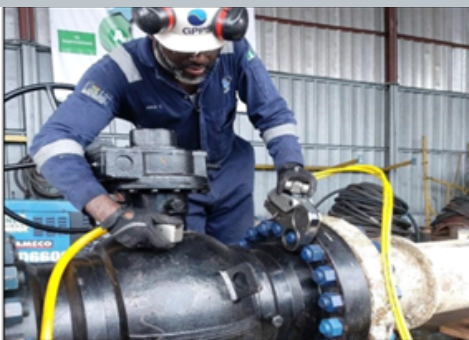
Flange management and bolting operation of Flow-line Valves
