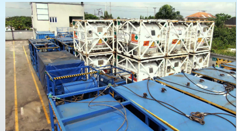
Liquid nitrogen tank of 2,000 USG capacity
